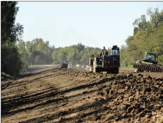
A Vicksburg crew constructs a section of levee Friday. Rain has put actual progress slightly behind scheduled progress. Work is expected to proceed rapidly with the dry weather, and the crew is expected to meet the scheduled completion date here for levee repairs, but additional work will continue after Oct. 9.
