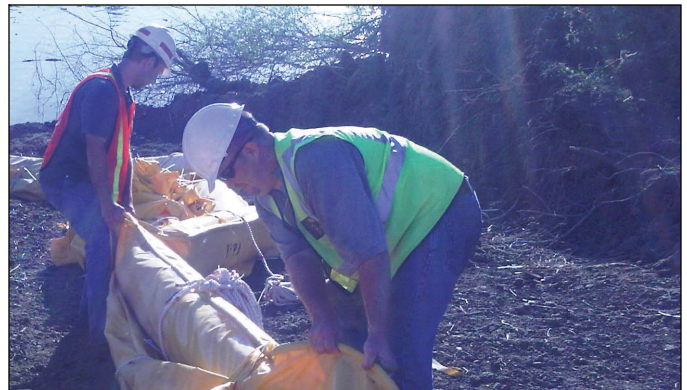
Engineers construct a silt curtain at the center crevasse Monday. The silt curtain will prevent silt plumes from entering the existing scour hole.
