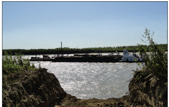
The dredge Iowa arrives Friday at the center crevasse. The dredge contractor is constructing a pipeline that will transport sand more than a mile from the dredge to fill the scour hole at this location.
