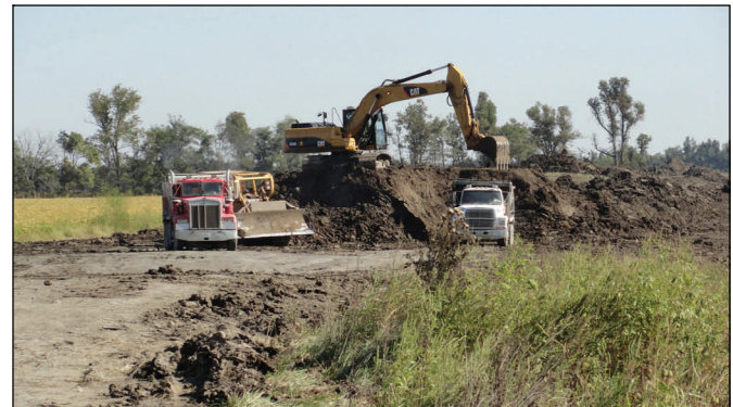
Clay is loaded into contracted trucks Thursday. The clay will be placed in the levee at the upper crevasse.
